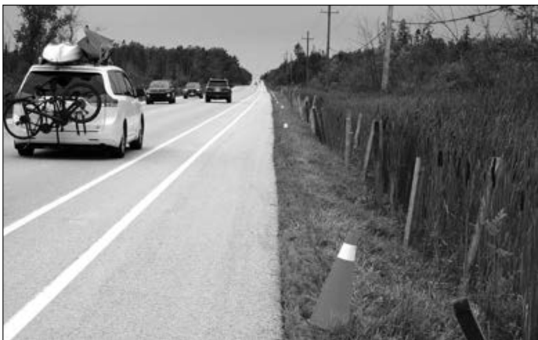
Photo: Fence posts are sitting in post holes along the shoulder of Highway 6 in the wetland area north of Cameron Lake Road. They will support wildlife fencing that will keep wetland creatures — turtles, snakes, frogs — off the highway.
