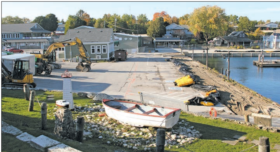
The head of Tobermory's Little Tub Harbour is fenced off while Fisheries and Oceans repairs the north and west walls of the harbour.
