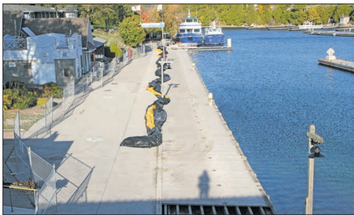
Photo: The recently (2009) repaired north wall of Little Tub Harbour will be reinforced to deal with a deteriorating wooden crib substructure.
