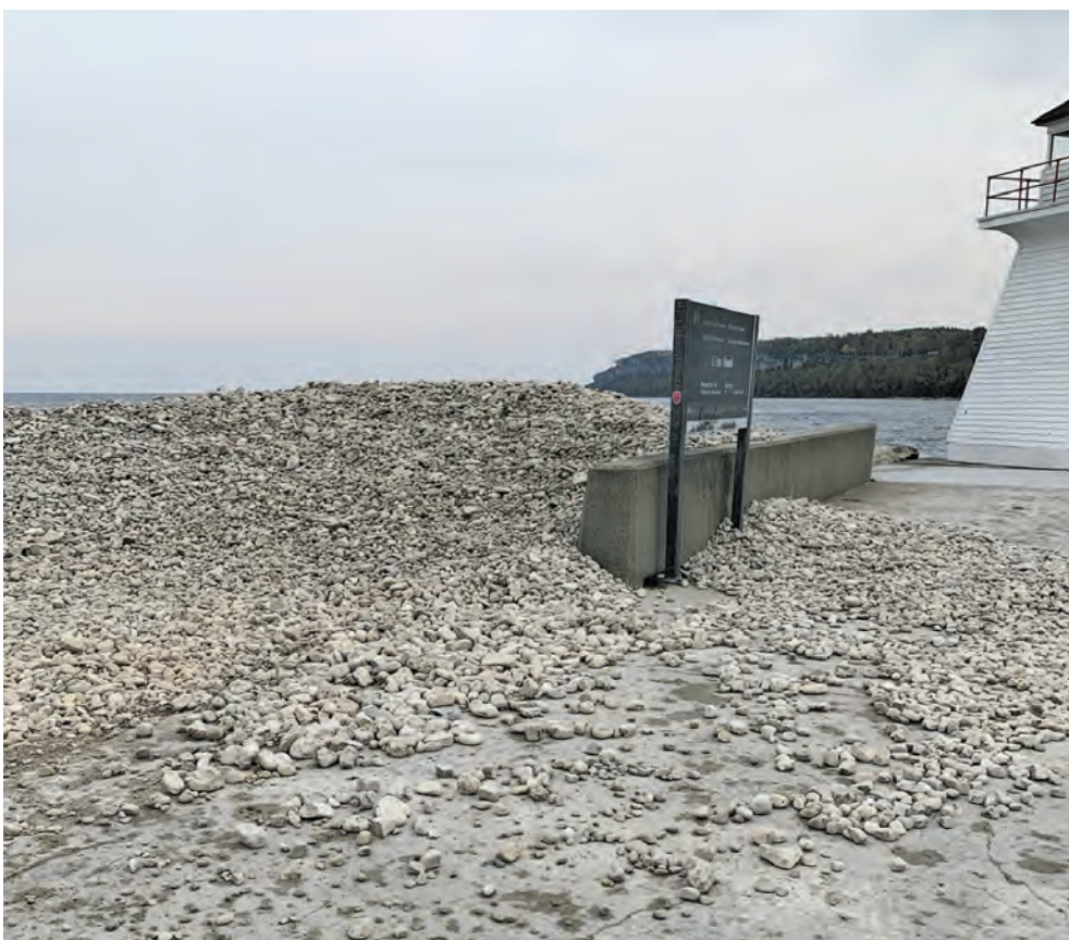
Photo Credit: Municipality of Northern Bruce Peninsula
