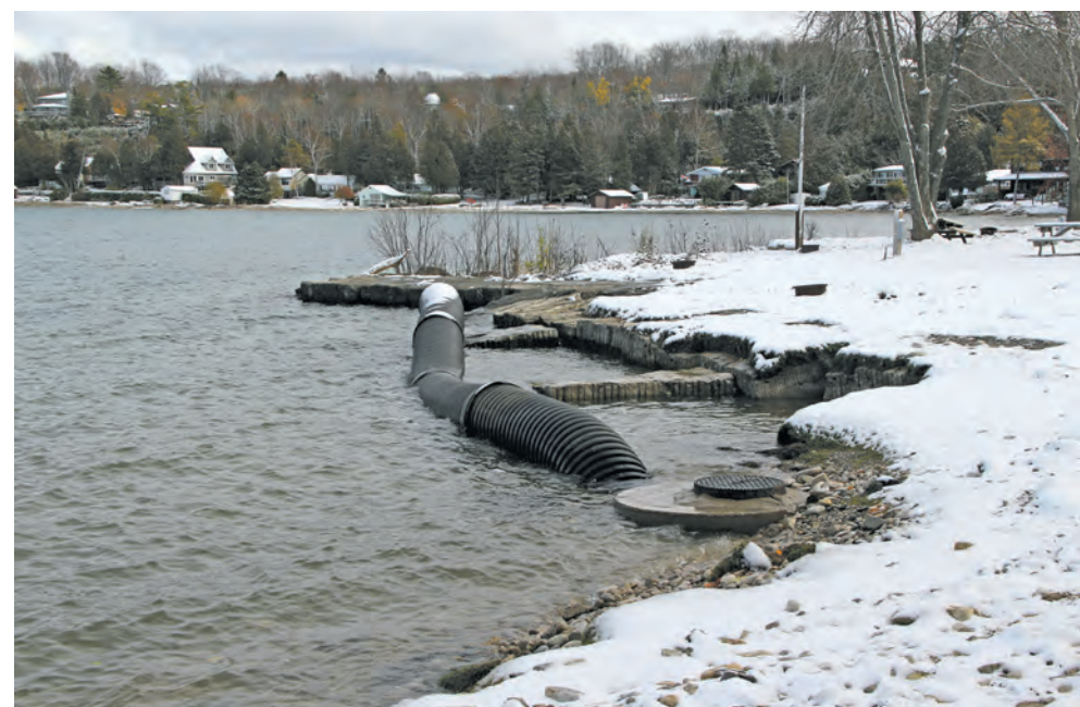
Photo: The shoreline at Lion's Head beach looking towards the campground after the storm.
