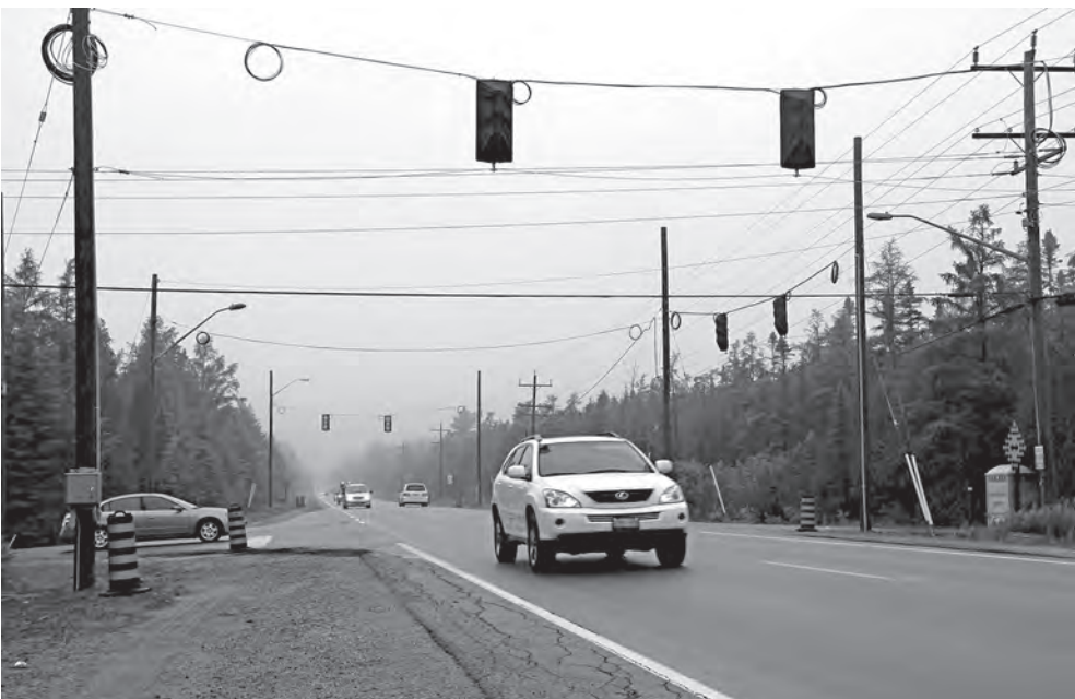
There are three sets of lights at the intersection of Hwy 6 and Dorcas Bay Road, but don't worry — they aren't permanent. They're only there to manage the lane closures while the culvert under the highway is upgraded.
